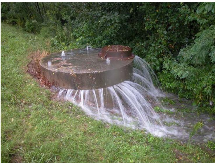
Elevated flows in the collection system can exceed the sewer main's capacity to get the sewage to the WWTP. When the sewer pipe capacities are exceeded, sewage may overflow at locations such as manholes, lift stations, and basements. These overflows and bypasses allow untreated sewage to bypass treatment, pollute the environ-
